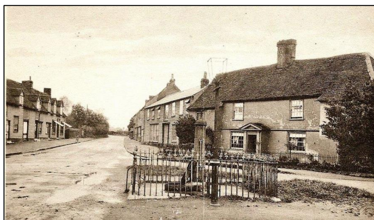
Figure 6: Hooks (later the Pump House)
